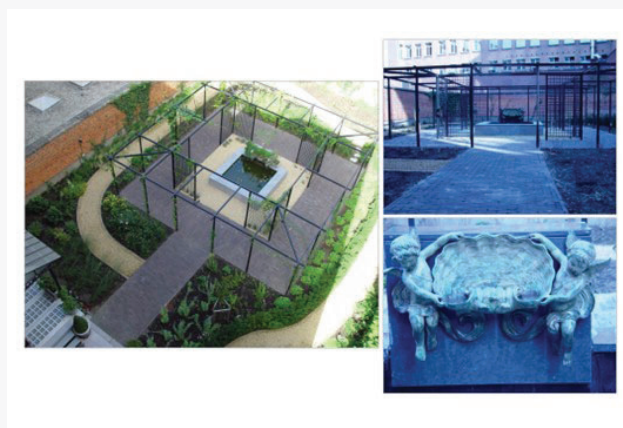
Figure 16: The garden of the building after the renovation in 2004
